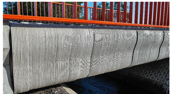
Figure 24.9 – 3-D Printed Bridge, Extrusion-based Technique 24.9
